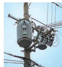
4 Pole-mounted transformer
