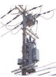
4 Step voltage regulator
