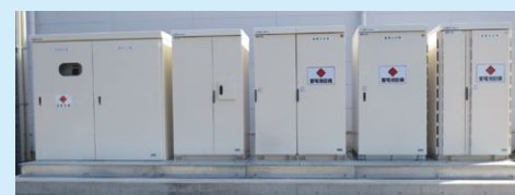
②-2 Storage battery system at the DAIHEN Technology Institute
