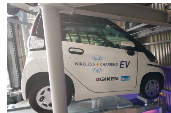
Wireless charging in the mechanical parking structure
