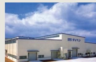
● Mie Business Office Manufacture of large-class power transformers
