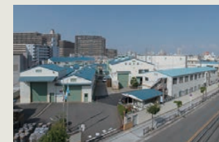
● Kanehira Plant Servicing of pole-mounted transformers
