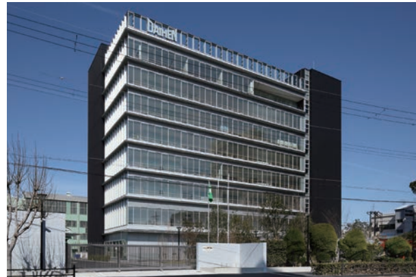
Head Office (Juso Business Office)
