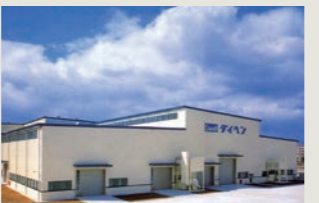
● Mie Business Office Manufacture of power transformers
