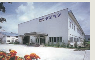
● Chitose Plant Manufacture of power transmission and distribution products
