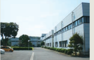
● DAIHEN Technology Institute Manufacture of clean transfer robots, dispersed power equipment, wireless power transfer systems, etc. Development of software.
