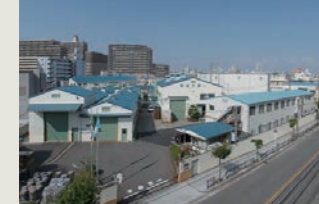
● Kanehira Plant Servicing of pole-mounted transformers
