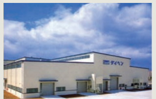
● Mie Business Office Manufacture of power transformers
