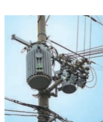
4 Pole-mounted transformer
