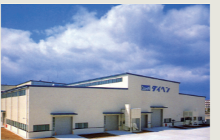
● Mie Business Office Manufacture of power transformers
