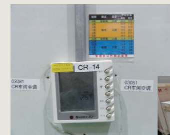
AC control panel (Temperature is set by managers.)
