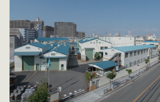
● Kanehira Plant Servicing of pole-mounted transformers
