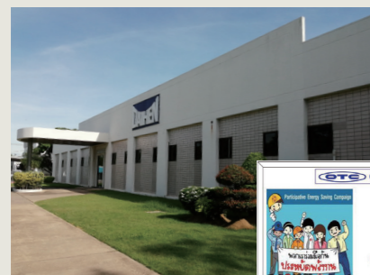
Company seen from the front
