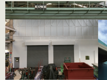
Thermally insulated wall seen from the outside
