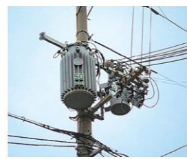
4 Pole-mounted transformer
